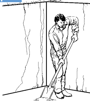
Utilize sand to level base of excavated area. Sand shall be compacted
