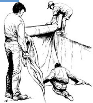
Lay geotextile (lay polypropylene liner if a Rainwater Tank is desired) along base and walls of excavated area.
