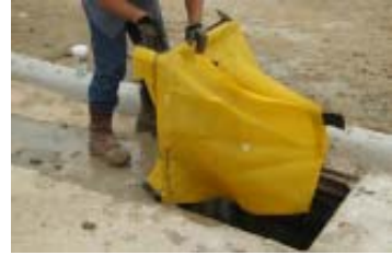
Slide Siltsack® over opposite side of grate.
