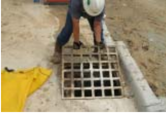
Remove grate from catch basin.
