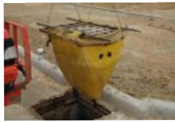
Removed Siltsack® is now ready for cleanout.
