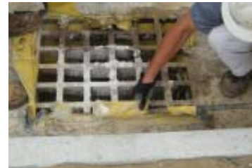
To remove Siltsack®, clean area around grate and slide rebar through Siltsack® pockets.
