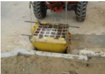
Slowly remove Siltsack® from inlet.
