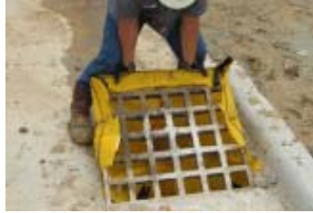
Slide Siltsack® over one side of grate.
