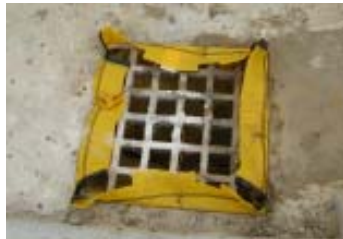
Installed Siltsack®.
