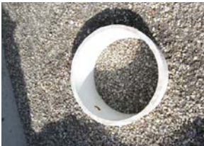
Figure 4: Pipe Installed Into Media
