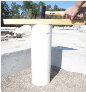
Figure 3: Hammer Pipe Into Media
